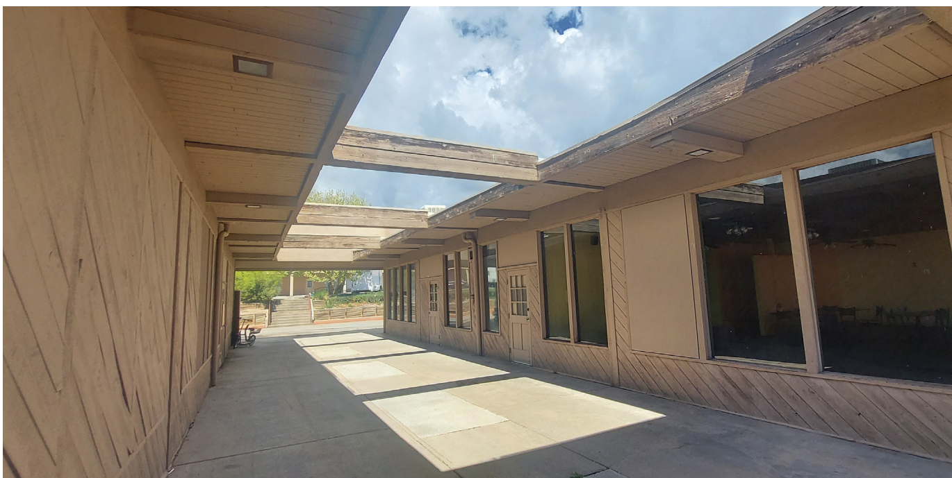
Figure 10. Entirely vacant building in the Mari Mac Shopping Center
