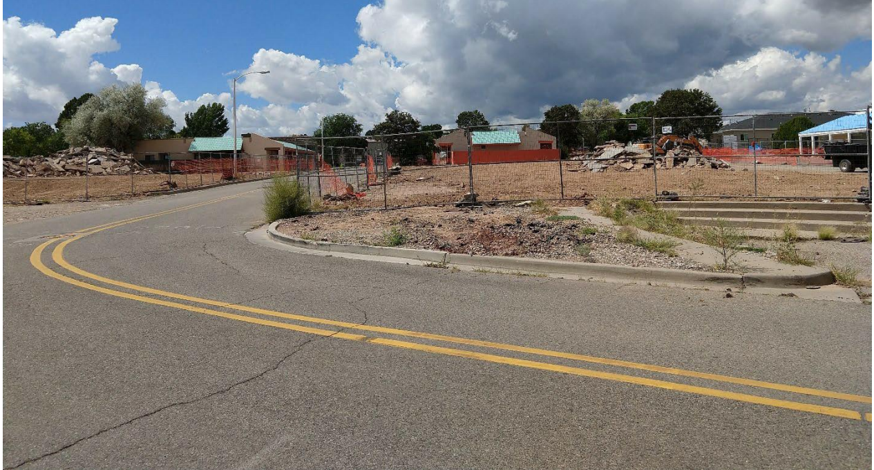
Figure 4. Recently demolished office building site along Longview Drive.
