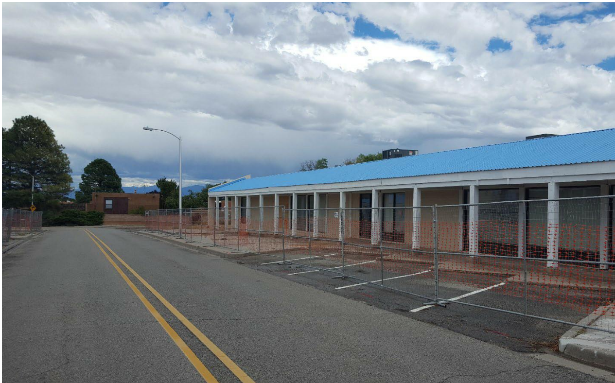
Figure 5. Office building along Longview Drive that was recently demolished due to multiple issues with the building.
